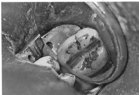
Fig. 5 Photograph shows tracing of the crack line to determine its extent. Methylene blue dye test was then used to soak the surface. Crack is visible in the center of the prepared groove
